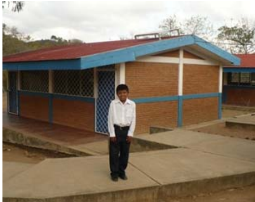
Sabana Grande elementary school building equipped with photovoltaic system.
